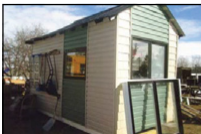
Custom Built 8'x16' Repair Shop recently sold for $2750
